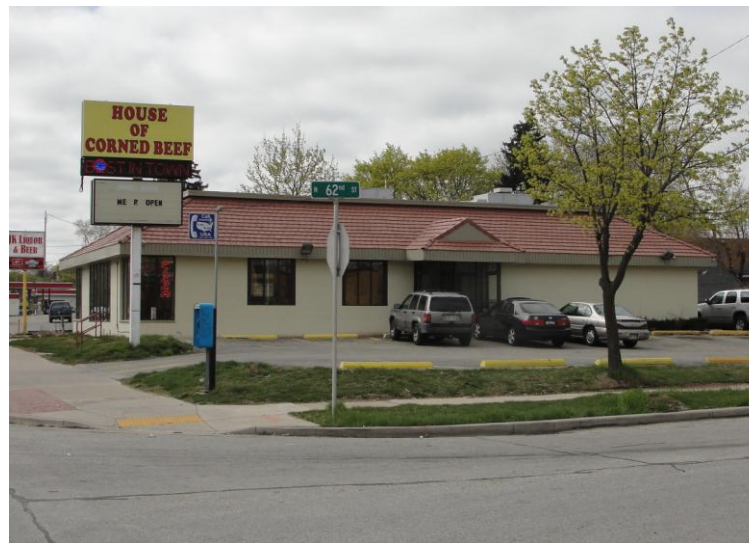
The same restaurant renovated and reopened. (6200 W. Silver Spring Dr.)
