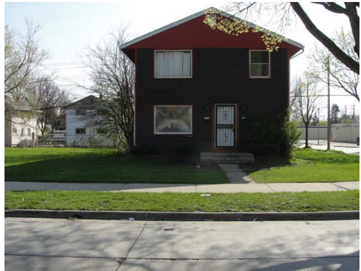
Current occupied and repaired home. (5640-5642 N. 62 nd St.).
