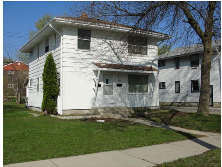
House currently occupied with repairs complete (5641-5643 N. 61 st St.).
